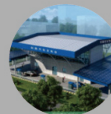
🔌 Solar, E-storage and charging solutions
